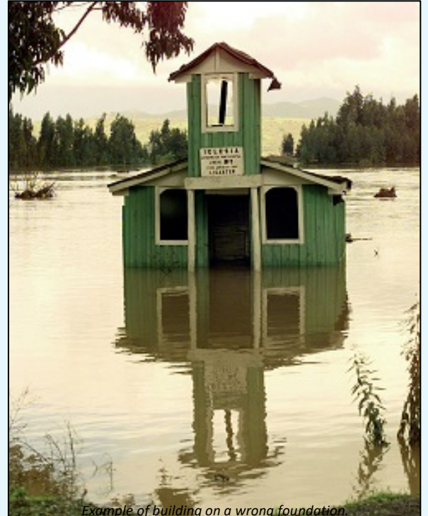
Example of building on a wrong foundation.
